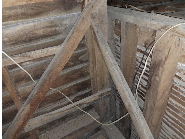
Upper right looks out over attic of our sanctuary.
